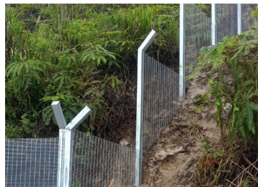
Post and mesh installation detail
