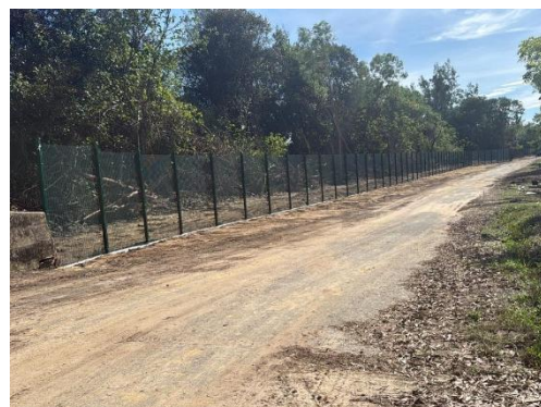
Anti-climb mesh and post installation
