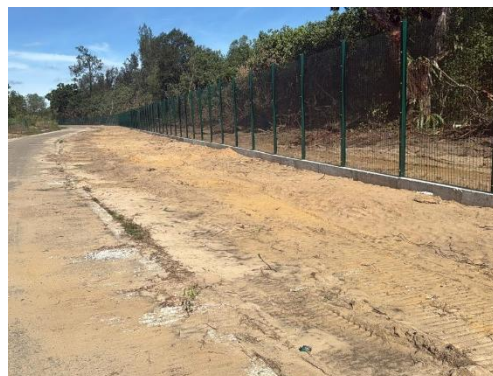
Perimeter following the forest boundary
