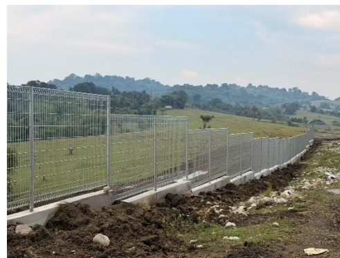
Fence line following the terrain
